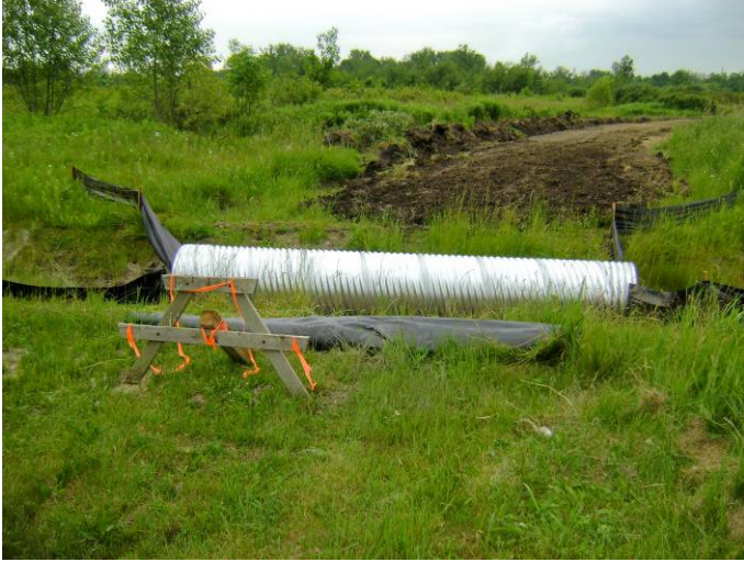
New conduit ready to cover for roadway
