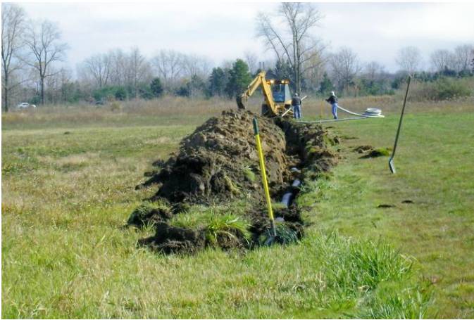
Trenching and laying the drainage tubing.
